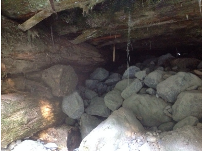
Right Bank Abutment when facing downstream
