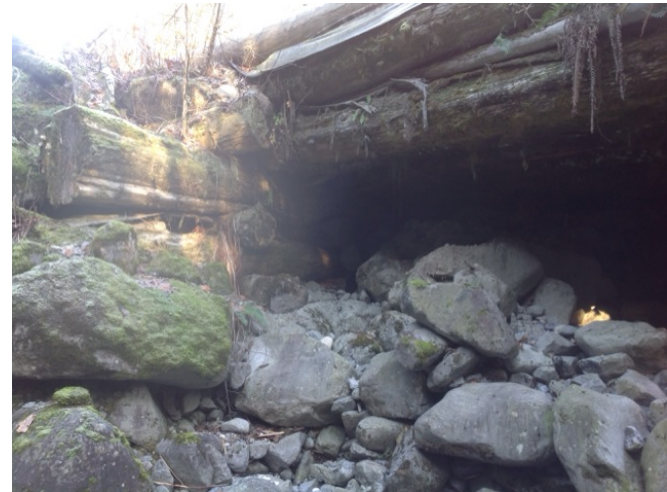
Right Bank Abutment when facing downstream
