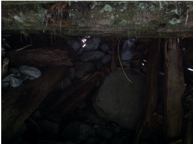
blocked portion of inlet viewed from under structure
