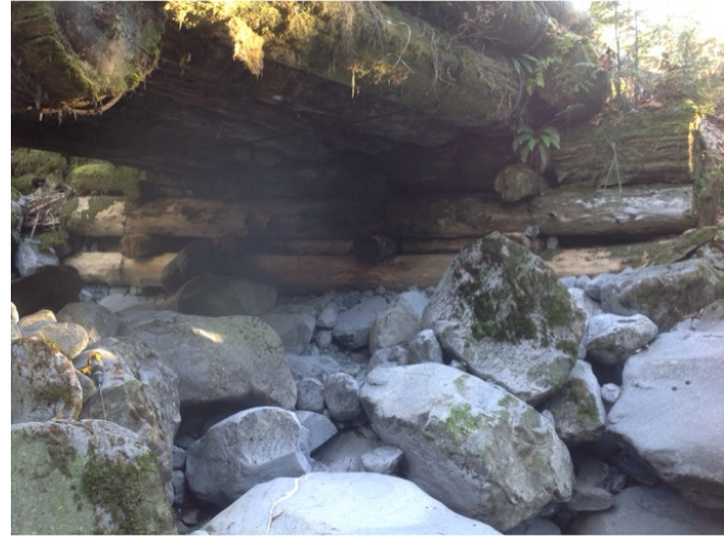
Left Bank Abutment when facing downstream
